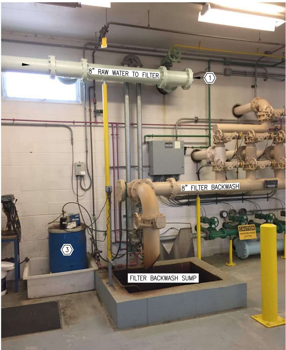
DUALATOR FILTER PIPING PHOTO NO.1 NO SCALE
